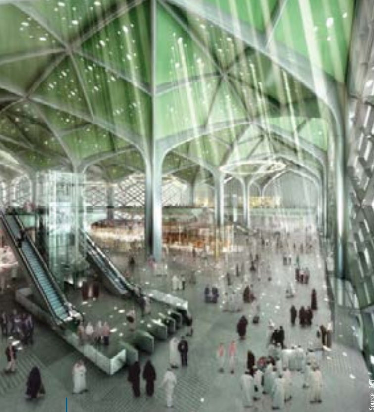
This rendering shows the interior of the Medinah station on the Haramain high-speed rail line project in Saudi Arabia. The tent-like canopy roof, pierced with small round windows, was assembled from modular, structural composite roofing panels, designed and fabricated by Premier Composites Technologies (PCT, Dubai, U.A.E.). ■
